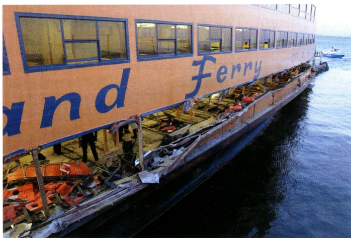
Damage to the M/V Andrew J. Barberi after it allided with a maintenance pier in October 2003.
