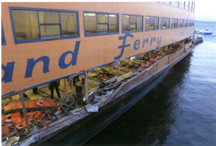
Left: Damage to the M/V Andrew J. Barberi after it allided with a maintenance pier in October 2003.
